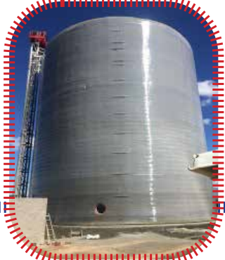
Brine Water Tank
